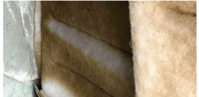
Figure 76. Dirty air filters
